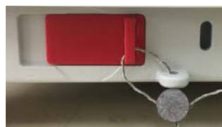
Locked with Wire Seal
